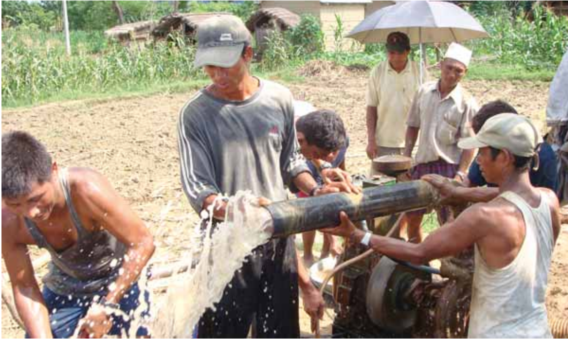
Checking the water flow of shallow tube well after its installation
