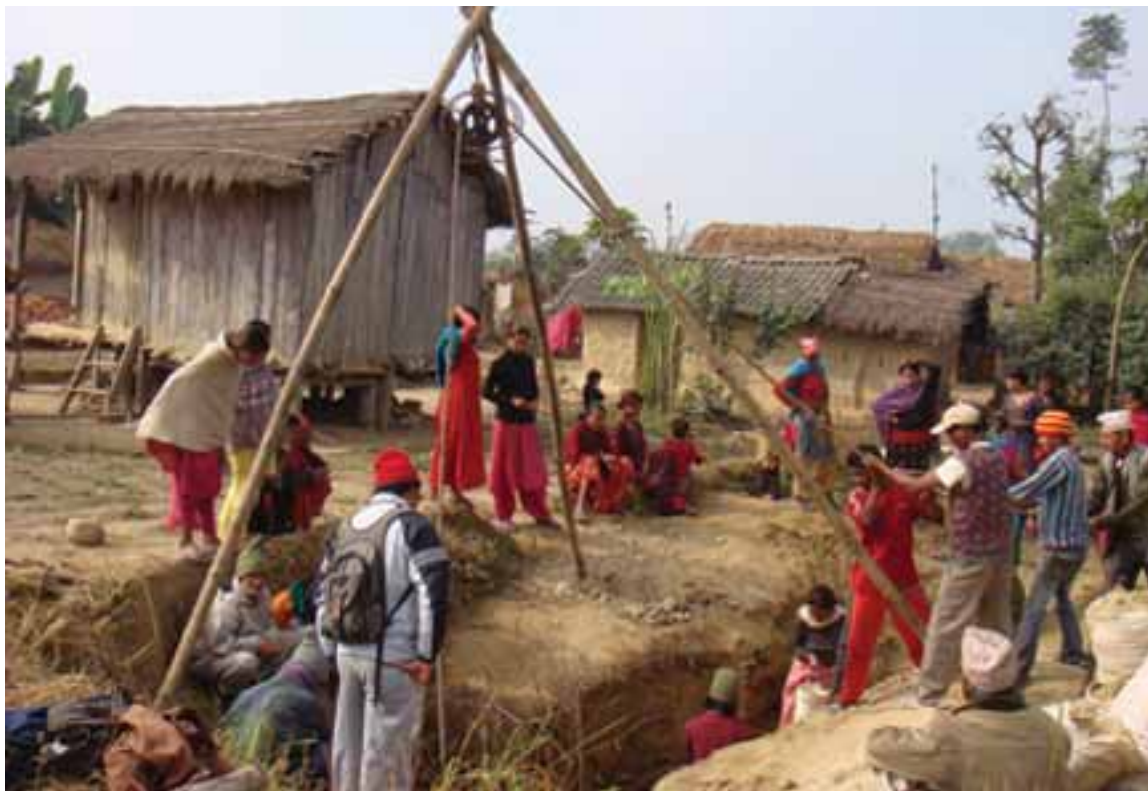
Communities installing shallow tube well in Bote tol, Pragatinagar, Nawalparasi
