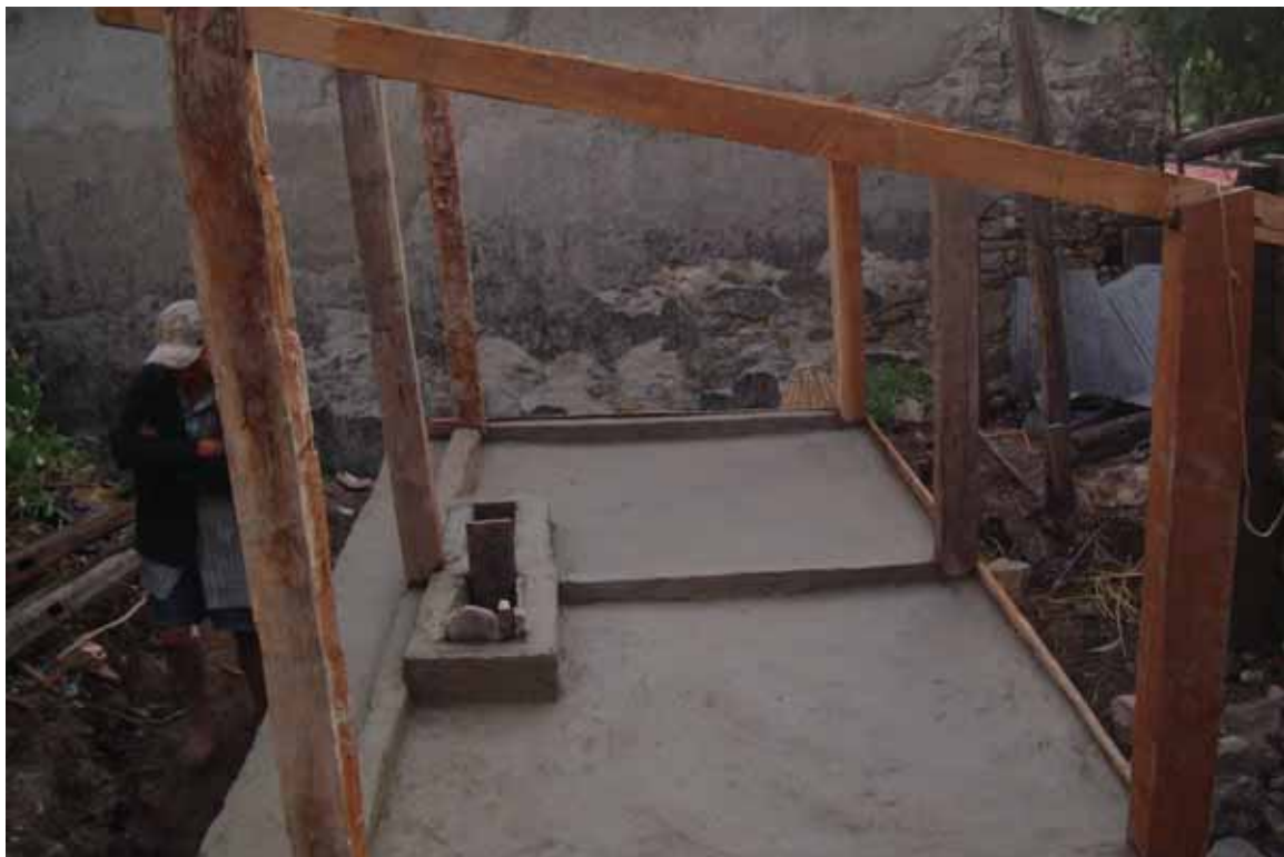
A model pigsty under construction
